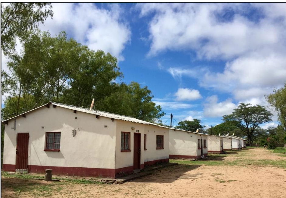
Figure 4: Onsite shared teacher accommodation
